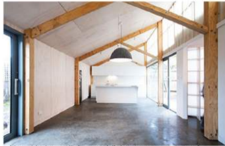
New kitchen, dining and living space, exposed structure: structural frame fabricated off site, and assembled on site in response to a very tight time frame specifically for this project.
